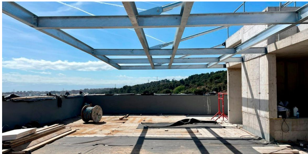
35 subsidised dwellings Molins de Rei (2022-under construction) Metronom
